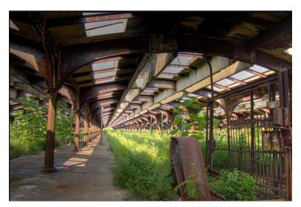
The Jersey City Bush shed was the largest ever built, at 308,000 square feet, slightly larger than the Toronto Union Station shed. Unlike Toronto, skylights were built over the platforms, part of the original Bush design, but eliminated in Toronto to reduce expenses. (photo by bridgepix)
