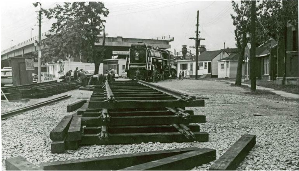
CNR 6213 begins its trip across the CNE grounds. It was taken to a siding beside the CNE by CNR S-13 no. 8513 and moved by a front-end loader onto the temporary panel track shown here. This was as far east as the Gardiner Expressway elevated section had been built as of this date. 10 August 1960. John D. Knowles photo.
