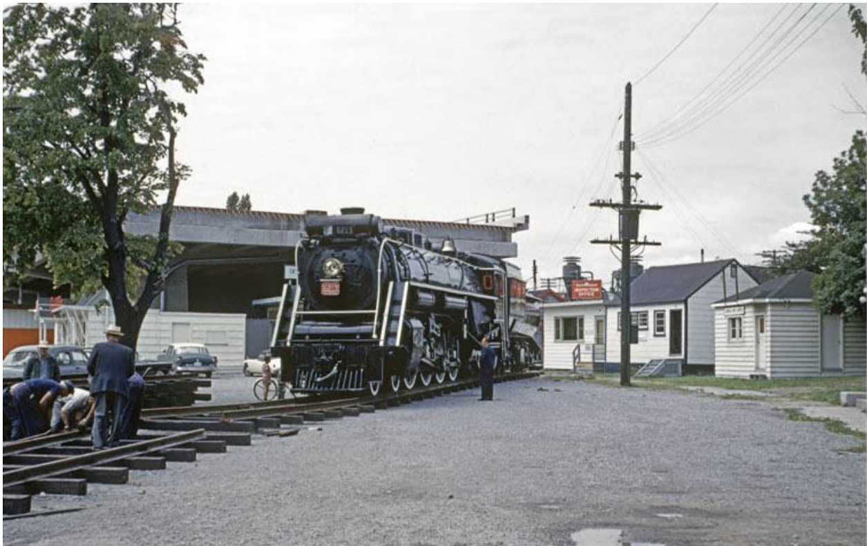
Workers lay a panel of track in front of 6213 as it slowly makes its way from its siding across to its berth beside Stanley Barracks on the south side of the CNE. 10 August 1960. John Mills photo
