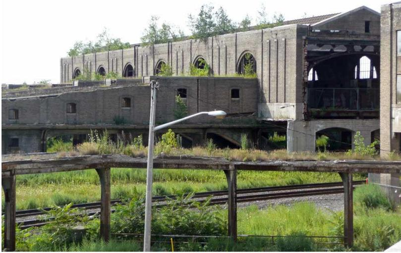
*The passenger concourse was built over the tracks, similar to VIA's Central Station in Montreal. In 1982, the concourse was partly demolished to permit Conrail double-stack freight trains to pass through the station complex.*
