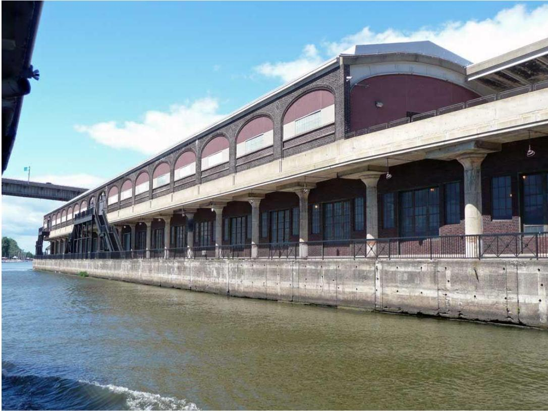
*The east end of the train shed from the Buffalo River. This was also a Bush train shed built on top of the freight shed which was underneath.*
