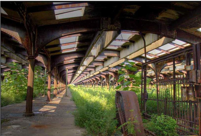
*The Jersey City Bush shed was the largest ever built, at 308,000 square feet, slightly larger than the Toronto Union Station shed. Unlike Toronto, skylights were built over the platforms, part of the original Bush design, but eliminated in Toronto to reduce expenses. (photo by bridgepix)*
